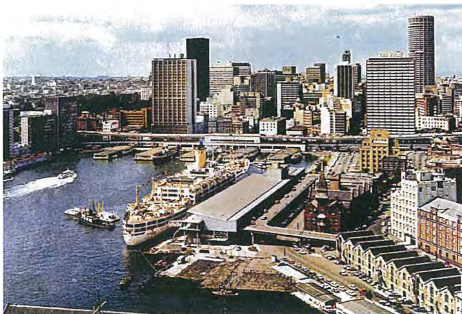
Figure 6.11 Circular Quay looking south in 1966 following the completion of Gold Fields House. The AMP tower and Gold Fields House act as bookends for the quay. (Source: City of Sydney Archives)
