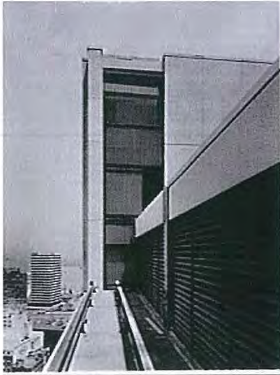
Figure 6.10 The modernist city, the air conditioning louvers on Gold Fields House demonstrating the new, sleek skyscraper design. (Source: City of Sydney Archives)
